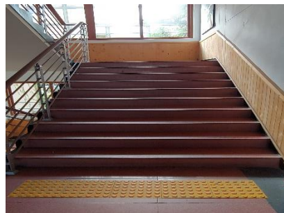
Figure. 2. Stairs in the target building.
