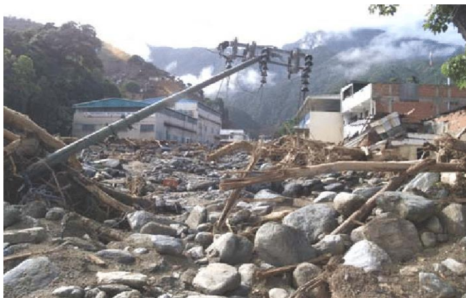
Figure 2-Image of debris flow damage (Schuster and Highland, 2007)
