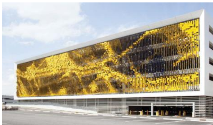
Figure 4: View of the parking lot of Ashkenazi Hospital / Rob Lee Studio
