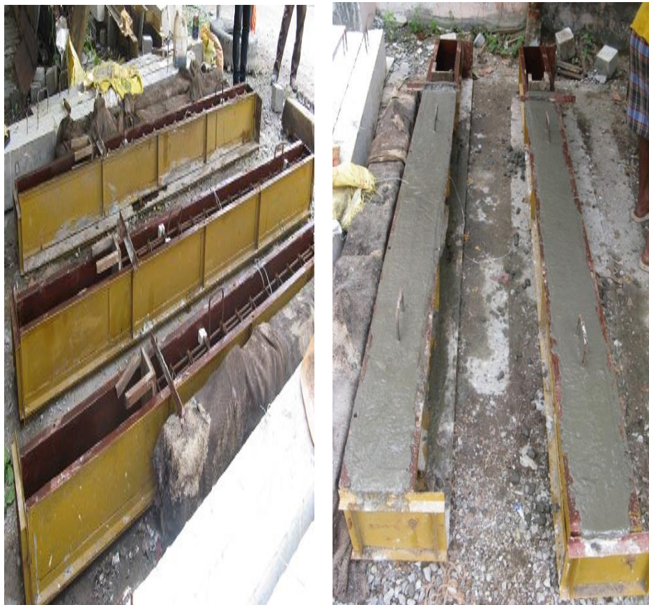
Figure 7: Mould and casting of beams
