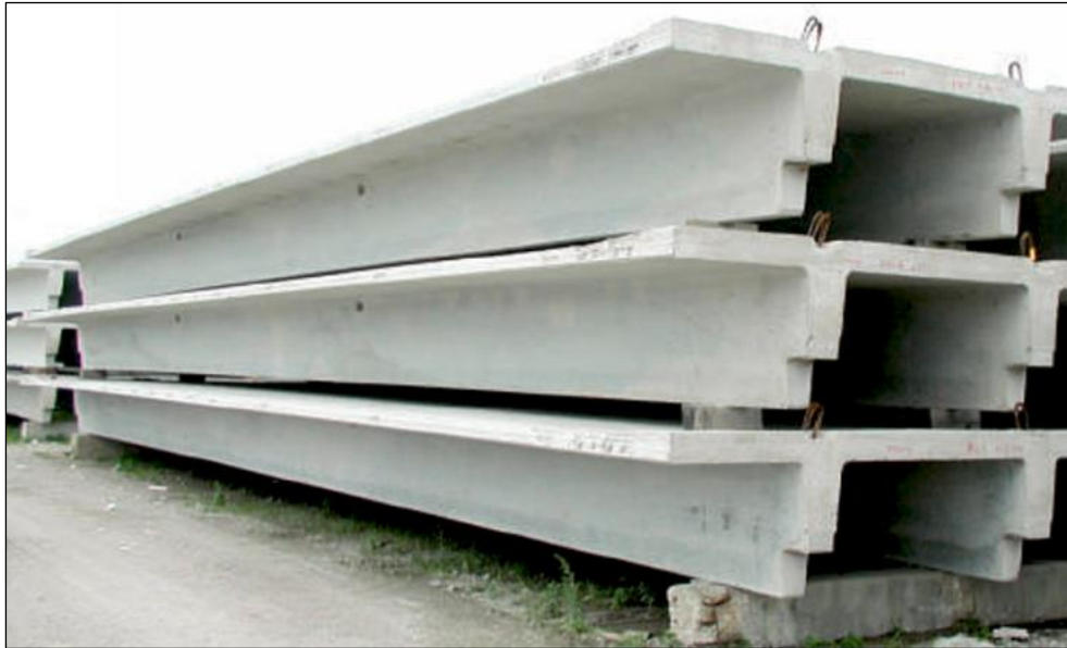
Figure 5: Stacking of DT members at storage yard (PCI Design Handbook, 2017)
