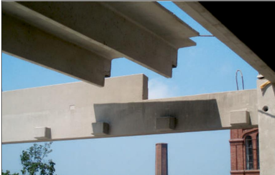
Figure 7: Erection of DT members at project site (PCI Design Handbook, 2017)
