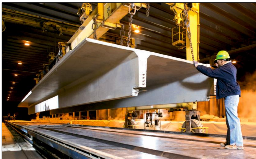
Figure 4: Stripping DT from long line casting bed (PCI Design Handbook, 2017)
