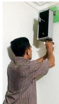
Pic 11. Speaker installation process for room acoustic system
