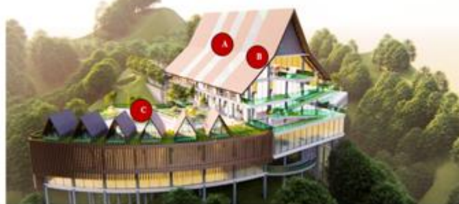
Figure.12(A) The roof system is used for natural lighting using sky light with stopsol glass material, (B) The roof covering uses single bitumen.(C) Roof garden system
