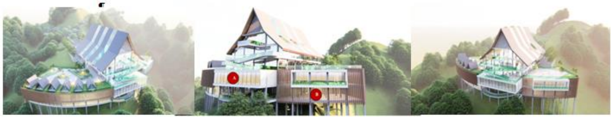
Figure.13 (A) The building facade system uses stained glass which reduces heat, (B) The vertical facade system uses aerobrise systems that regulate the opening for air.
