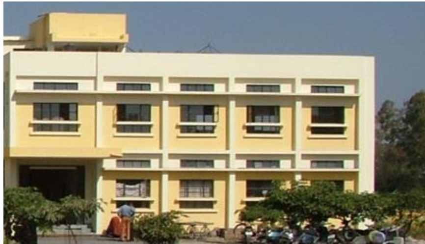
Figure 4 View showing overhang and window details
