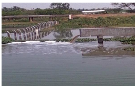
Fig3: Sewage Treatment plant.
