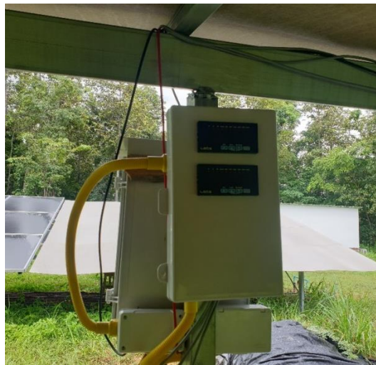
Fig.8 Installation of the meter
