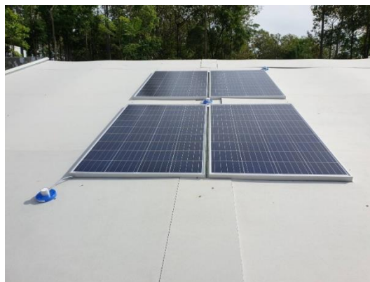
Fig.6 Installation of PV reference cell
