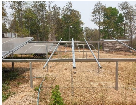
Fig.2 INSTALLATION OF PV SYSTEM STRUCTURE
