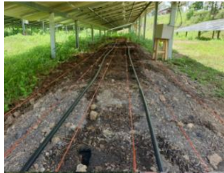
Fig.9 Installation of irrigation system
