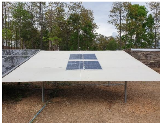
Fig.3 Installation of PV panel and smart board
