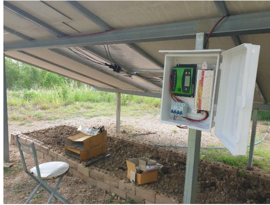
Fig.4 Installation of the control box and cable connection
