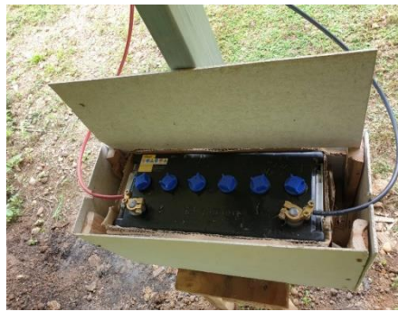
Fig.5 Installation of the battery
