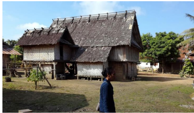
Figure 3 Tai-Lue house in Baan Na Yang Tai, Nam Bak, Luang Prabang Province Lao People's Democratic Republic
