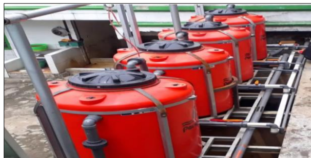
Fig 10. Piping installation process
