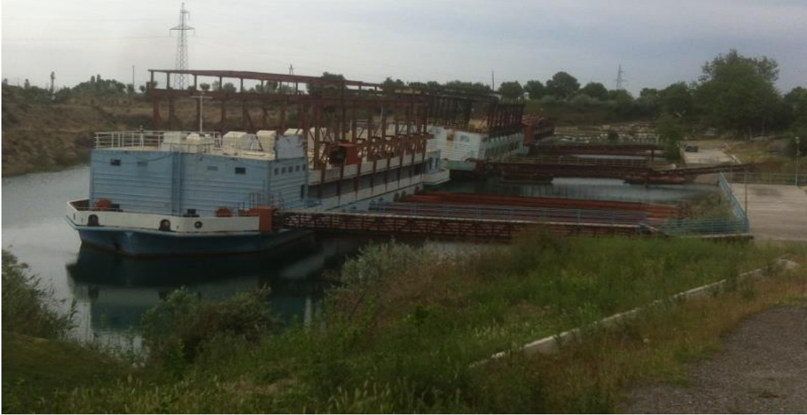
Figure 1. Khoja Bakyrghan – 1 pumping station
