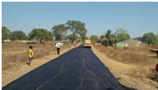
Fig 1.1 Construction of SDBC pavement
