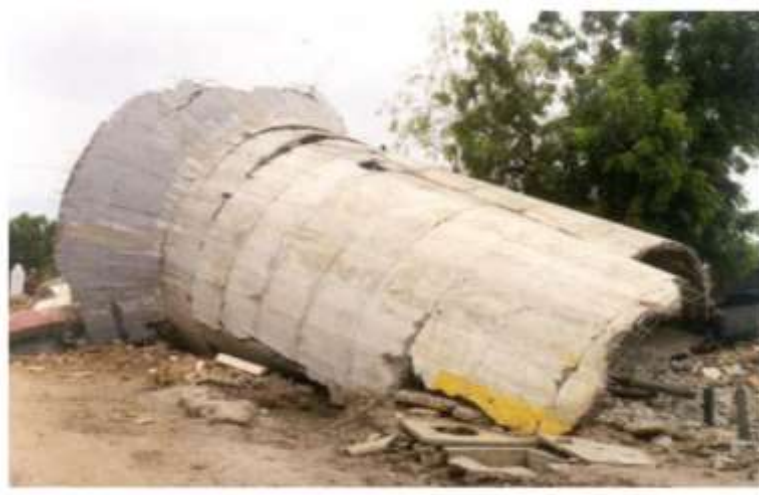
Fig 1: Failure of elevated Water Tank
