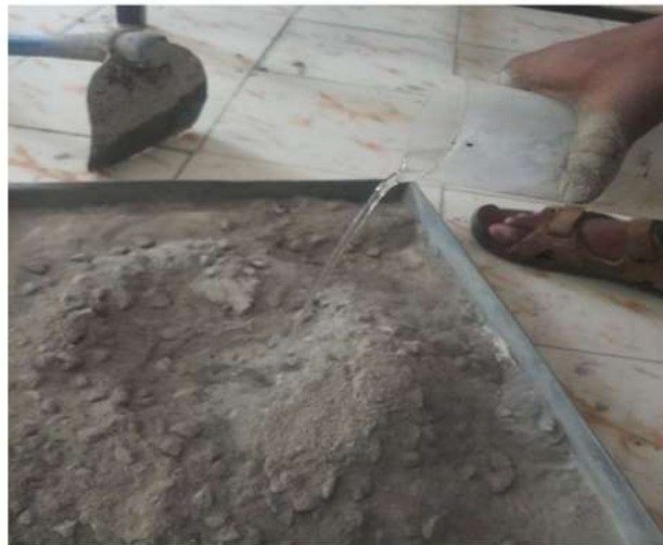
Fig. 4: Mixing of Concrete
