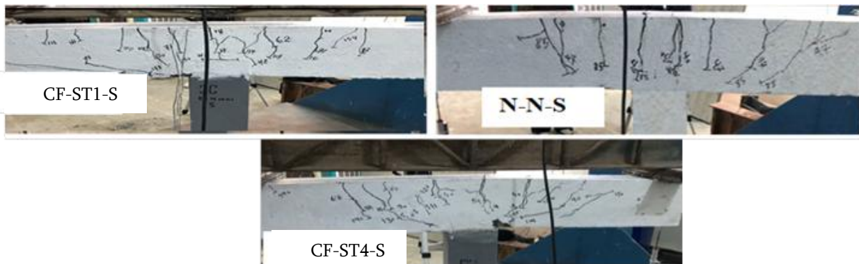
Figure 10. showing the cracking pattern of the tested specimens
