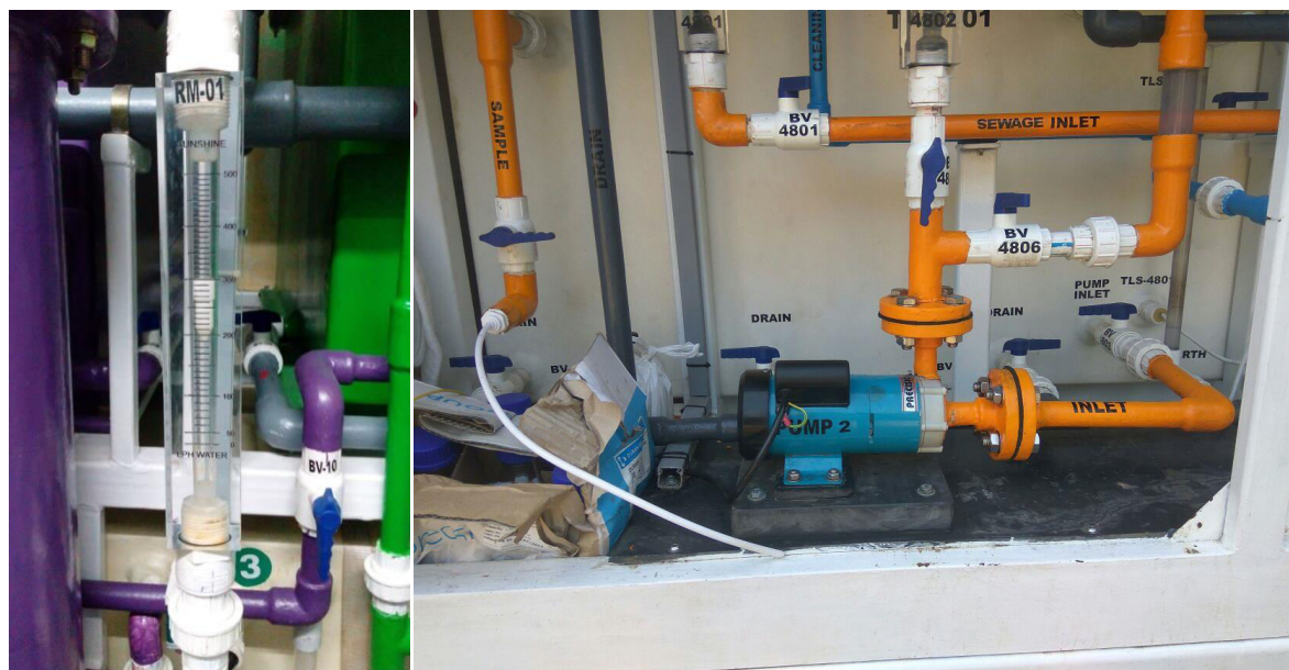
Fig.4 Level Indication system & Fig.5 Flow pipeline system
