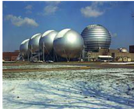
Figure 3: Langley indraft supersonic wind tunnel vacuum sphere
